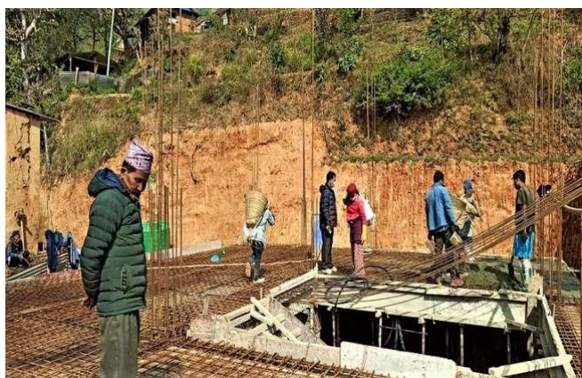
Figure 30: 1 st floor roof slab casting in Janajagaran Basic School
