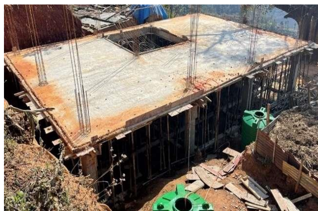
Figure 31: During monitoring after slab casting in Janajagaran basic School
